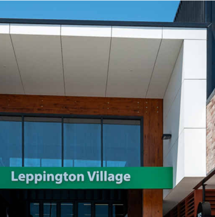
CODE: FC1 MATERIAL: FIBRE CEMENT CLADDING OR SIMILAR COLOUR: WHITE FINISH: PAINTED PANELS WITH EXPRESSED JOINTS
