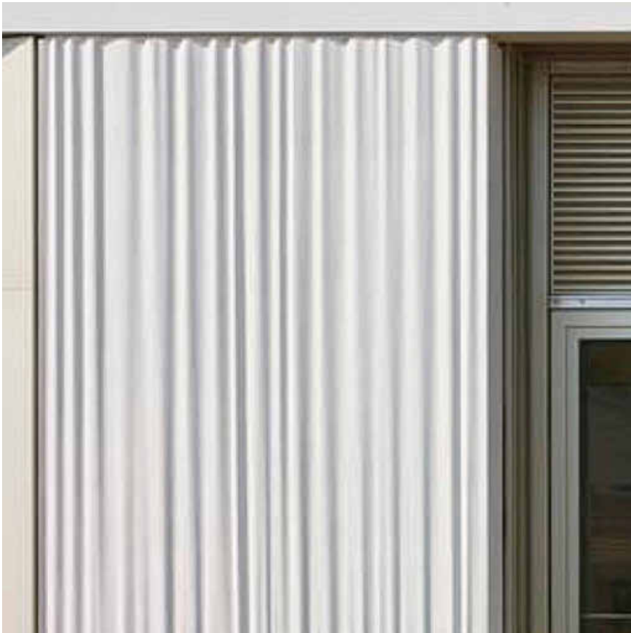
CODE: CP2 MATERIAL: PRECAST CONCRETE WALL PANELS COLOUR: PLAIN FINISH: PROFILED FORMLINER
